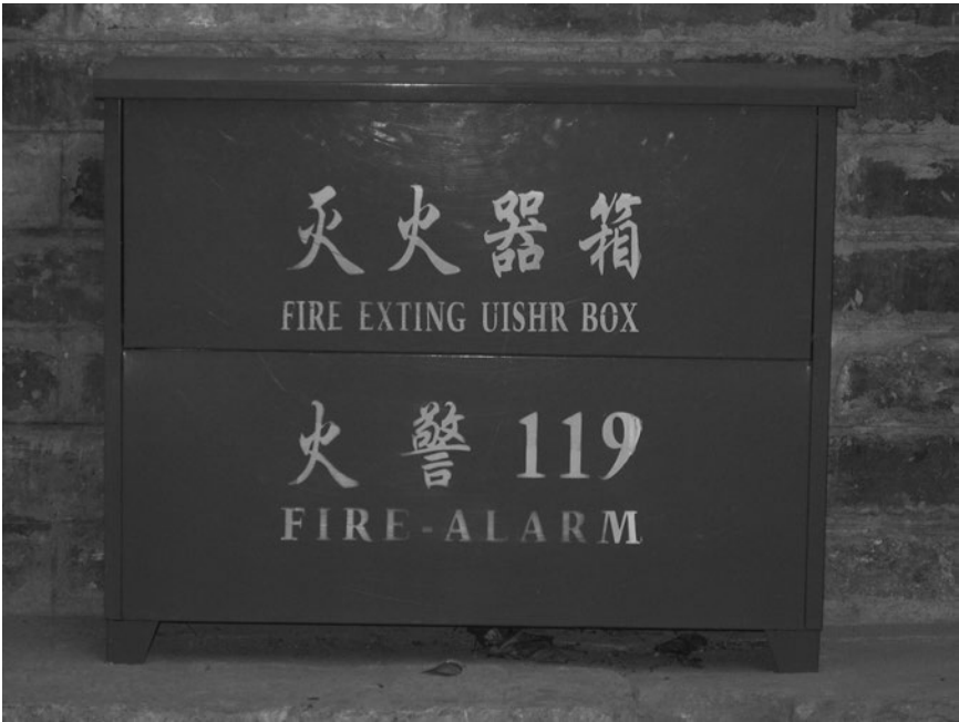
Figure 1.1 'Fire Exting Uishr Box'
