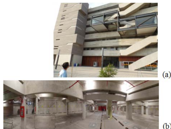
Figure 1. (a) New engineering building of the PUCP (b) Panoramic view of the basements
