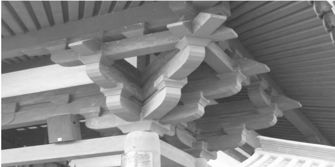
Figure 2. An example of dougong in traditional Chinese architecture. Source: Xinhuanet.
